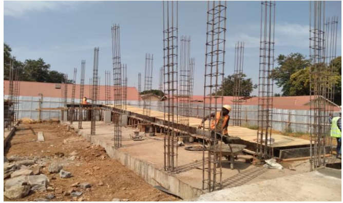
Figure 2 Ramp slab preparation
