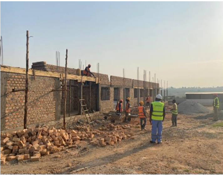
Works In Progress
