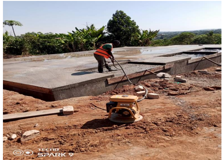
Foundation setup
