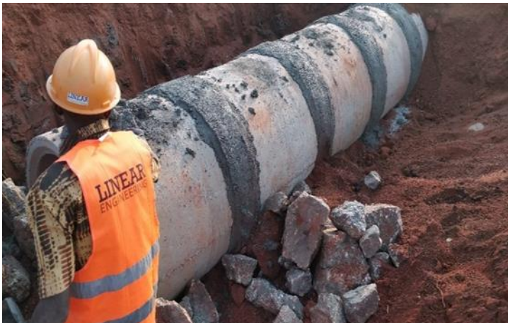
Culvert installation
