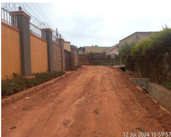
Shaping of the Road after drainage Construction
