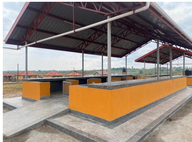
Completed market stalls
