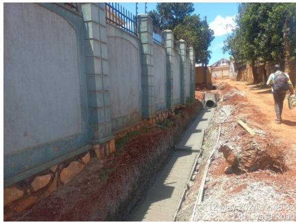
Casting of reinforced concrete base
