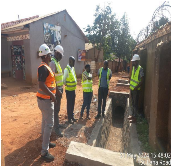
During site inspection
