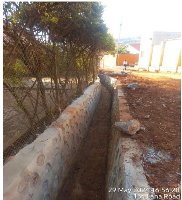
Stone pitching works
