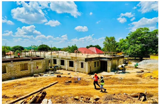
Figure 4 Slab curing and preparation
