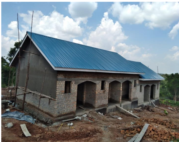
Plastering works in progress
