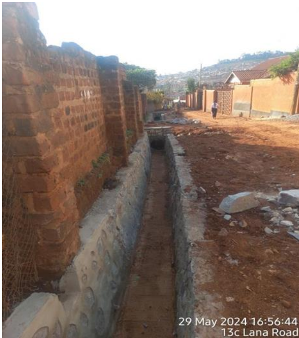
Stone pitching works
