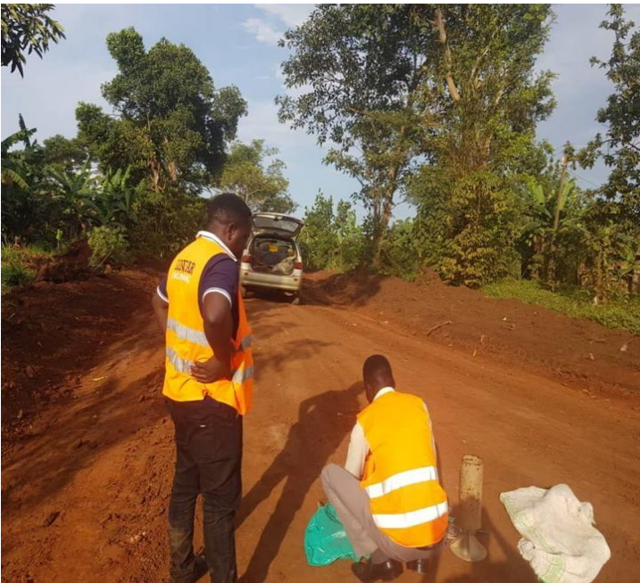
Road compaction tests
