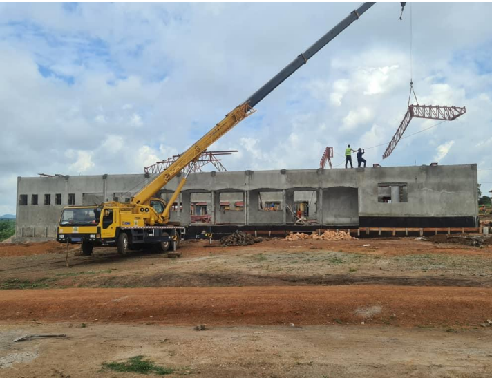
Roofing of community center in progress
