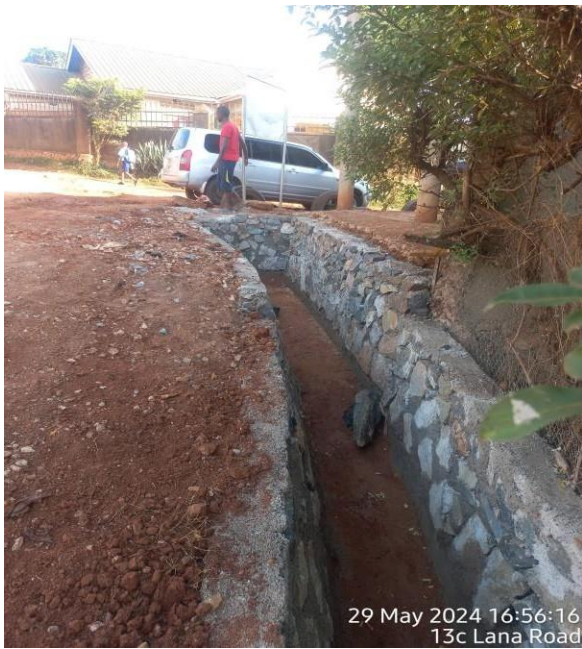
Stone pitching works
