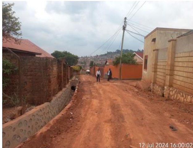
Shaping of the Road after drainage Construction
