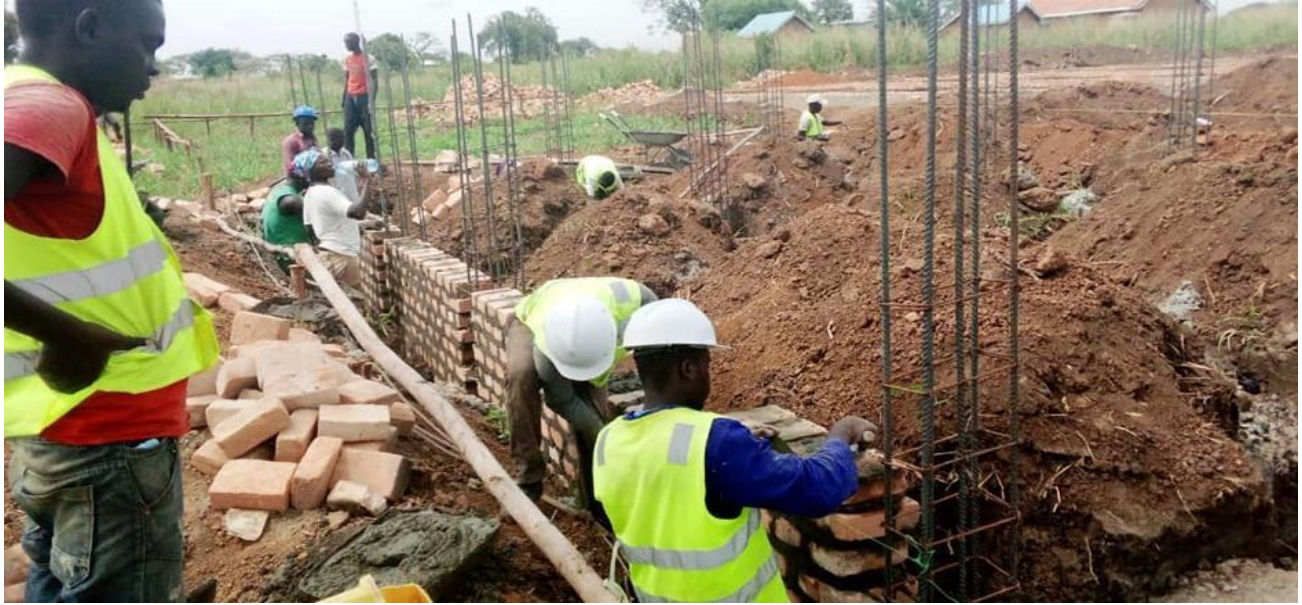
Plinth walling in progress
