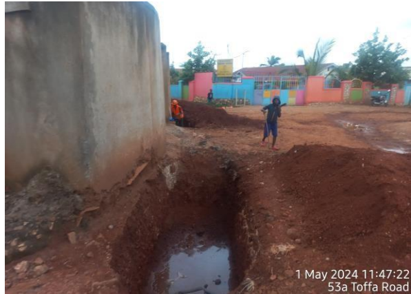
Excavation for drainage
