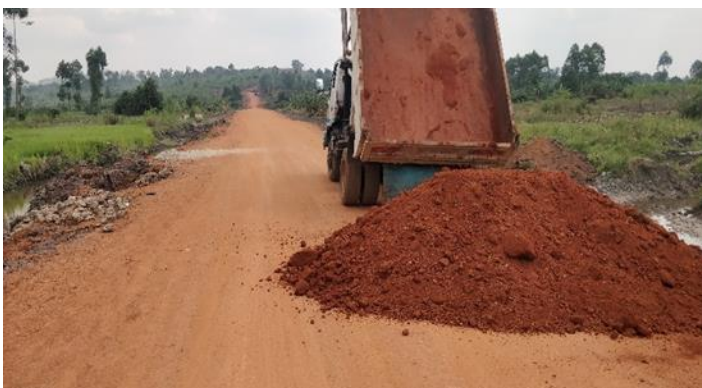
Murram dumping and spreading
