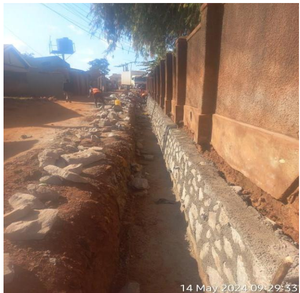
Stone pitching works
