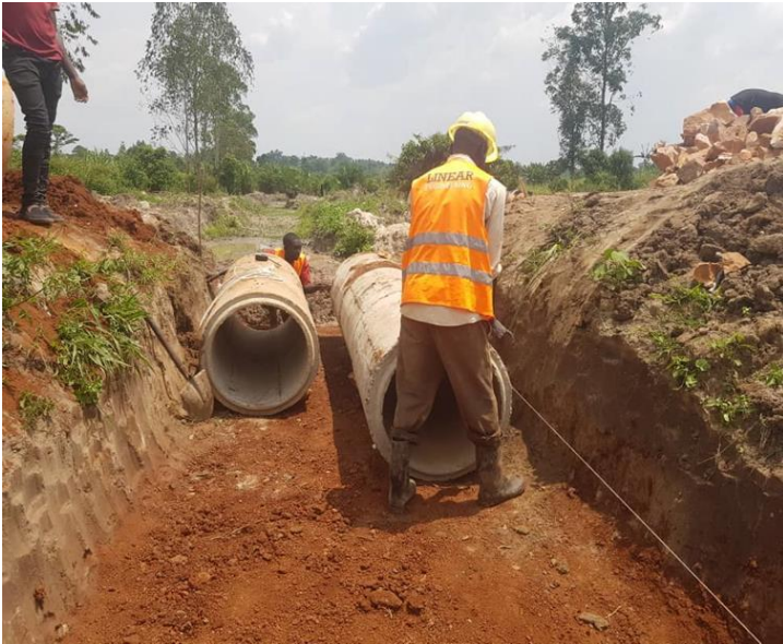
Culvert installation
