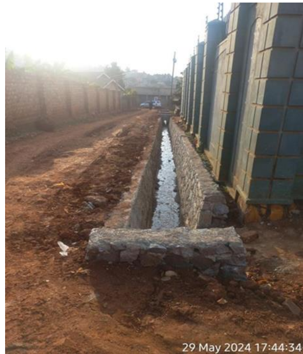
Stone pitching works
