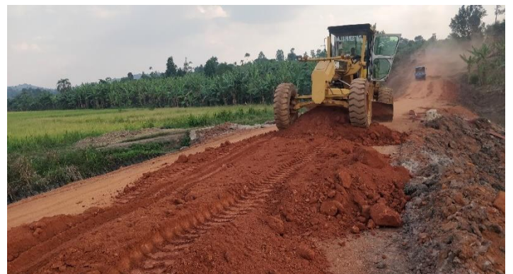
Murram dumping and spreading
