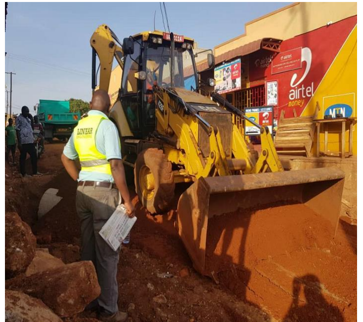
Works in progress
