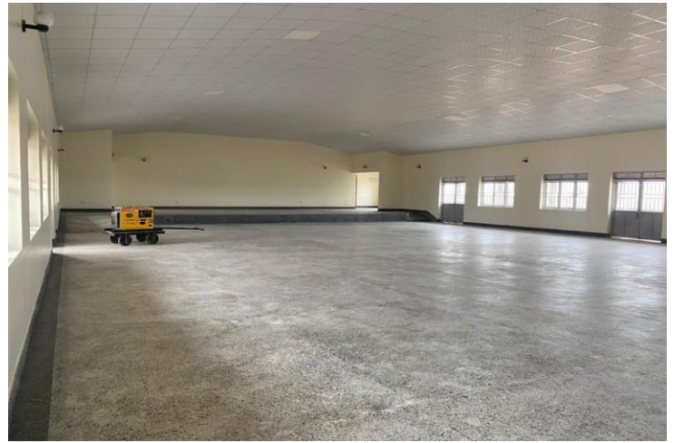
Interior view (Completed) of the Community center
