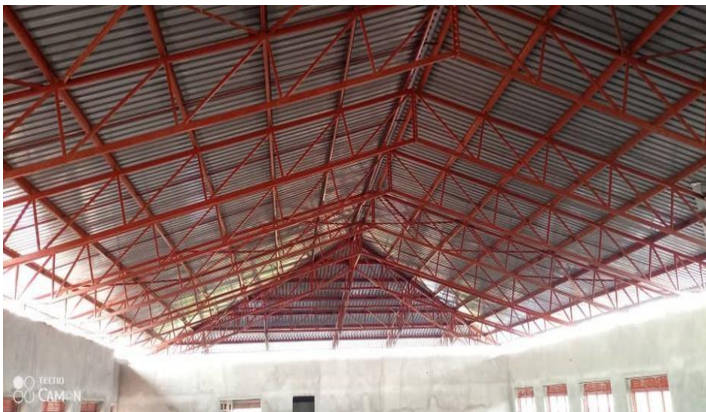
Roof truss (Interior)
