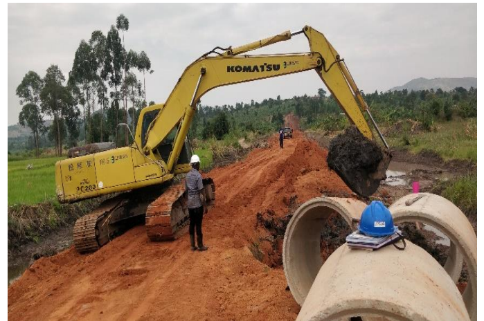
Culvert installation
