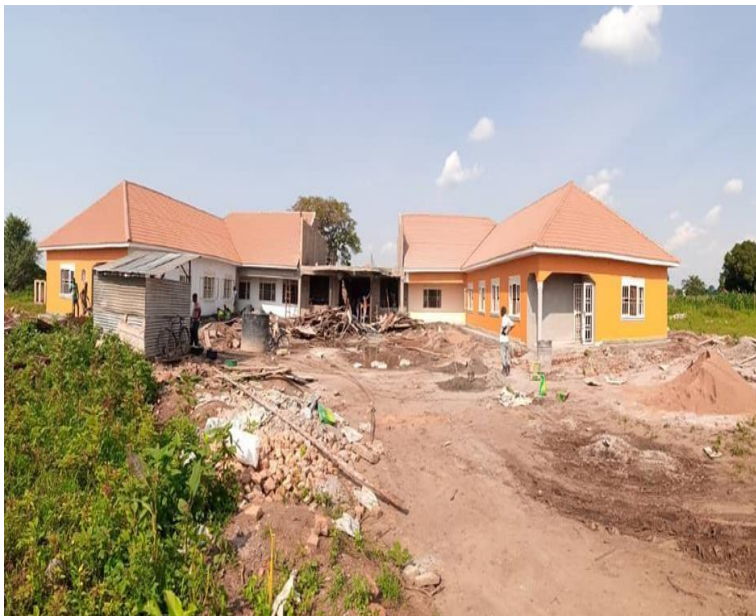
Figure 1 Works in Progress
