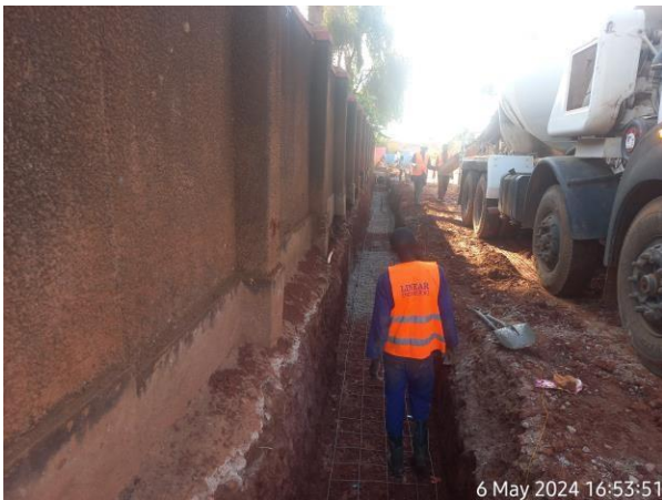
Casting of Reinforced Concrete base
