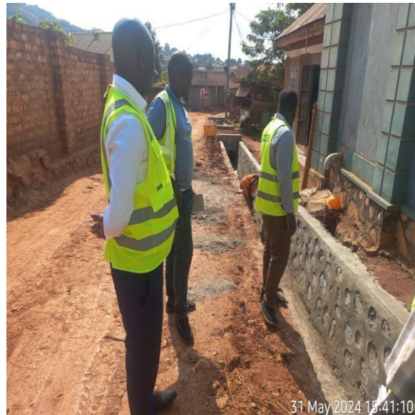
During site inspection
