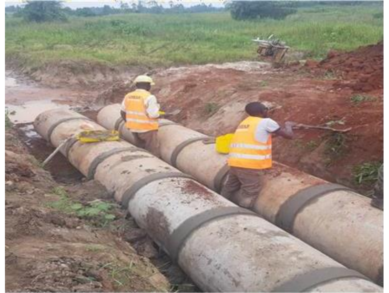
Culvert installation
