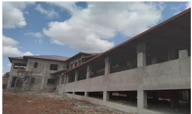
Figure 6 Plastering in progress
