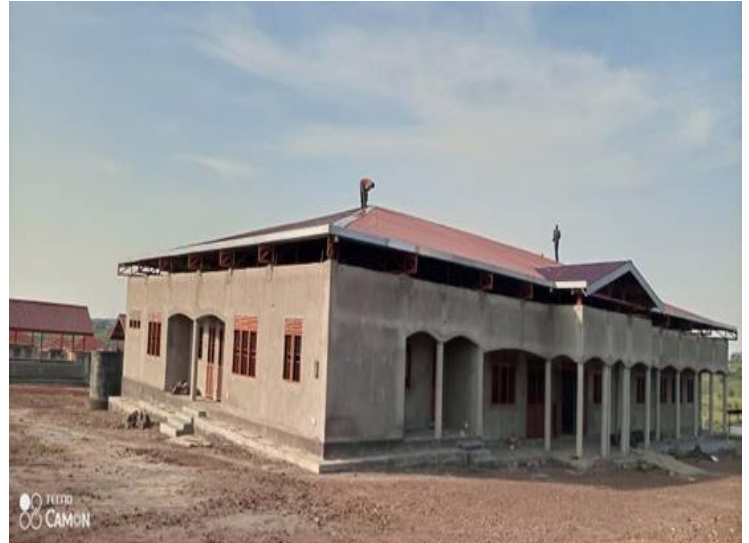
Front View of the roofed community center
