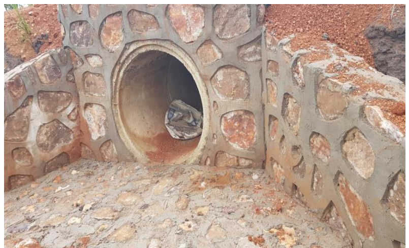
Installed culverts
