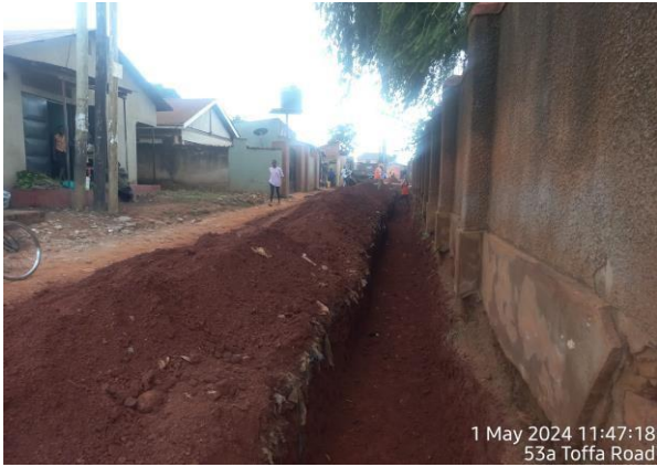
Excavation for Drainage
