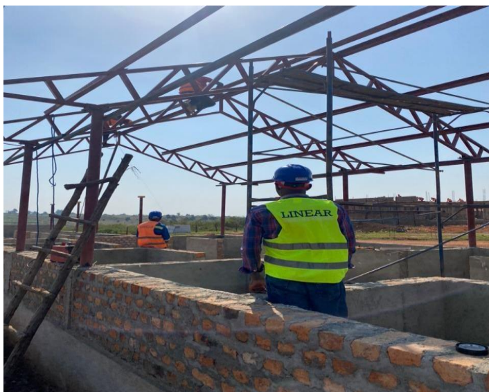
Roofing of market stalls
