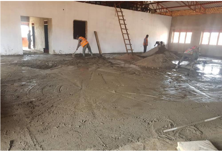
Interior works in progress-Community center
